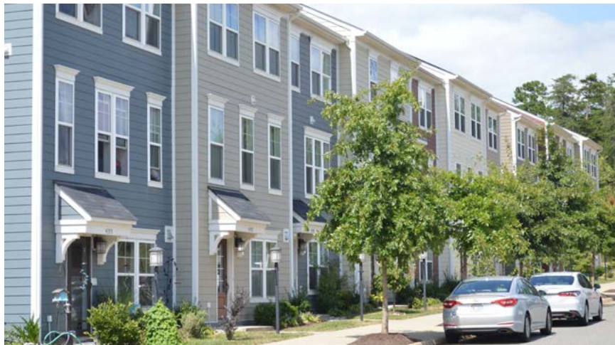
Community Design Guidelines provide criteria for the built environment during the review process for new development.
