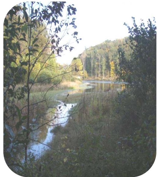
Lickinghole Sedimentation Basin
