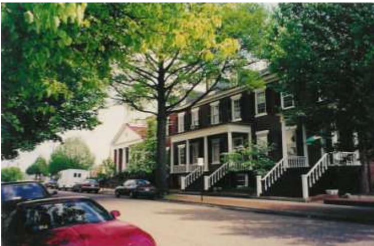
Figure 5.4. Example of a Residential Neighborhood Shown with onstreet parking & shallow front setbacks
