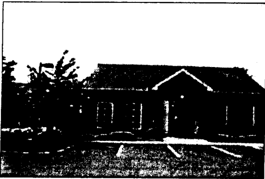
Wachovia Bank, Route 29N
