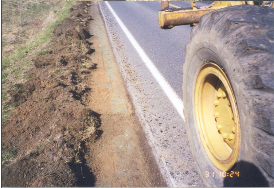
ATTACHMENT D - MOTOR-GRADER TRENCH WIDENING
