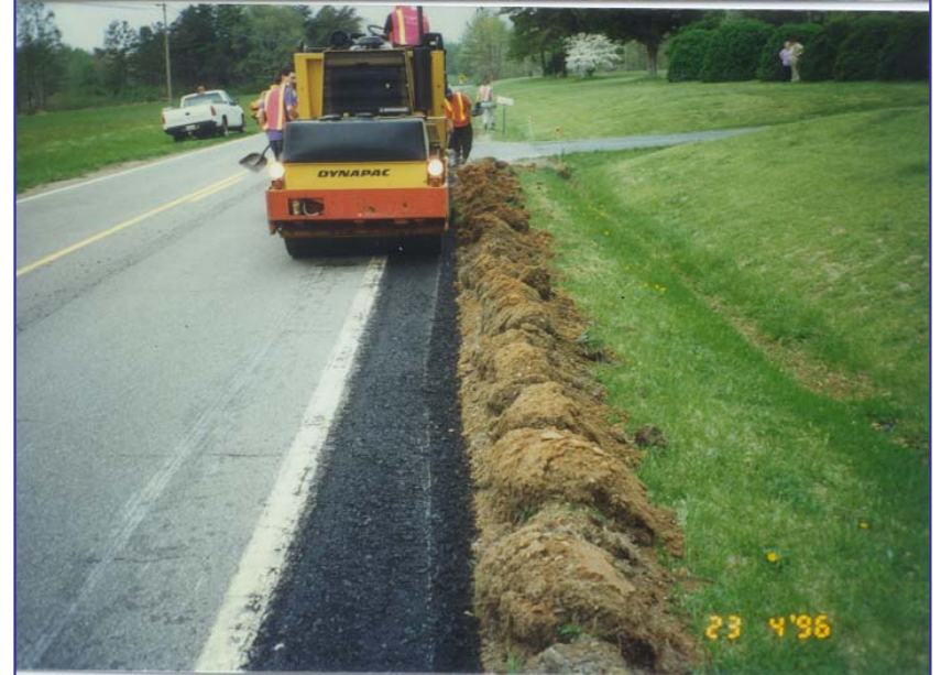
ATTACHMENT D - MOTOR-GRADER TRENCH WIDENING
