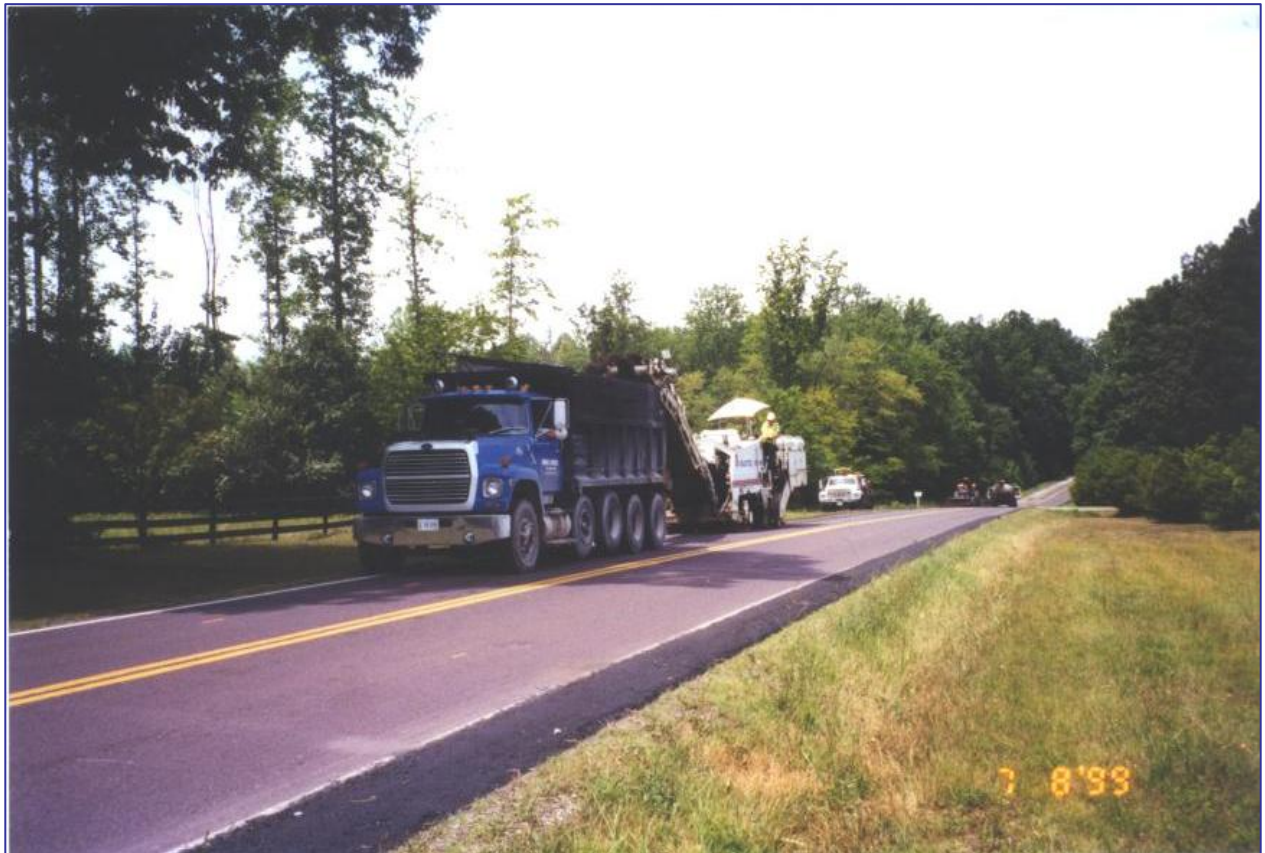
ATTACHMENT C - MILLING MACHINE TRENCH WIDENING
