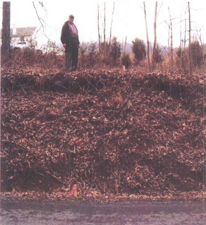
Bank along Craigs Store Road at location of proposed new entrance (see stakes), showing initial steep slope and rise to elevation of existing driveway (see truck at top left).
