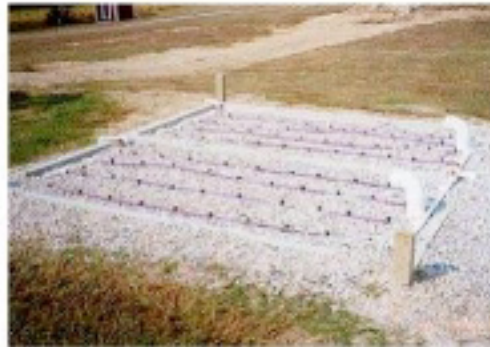
Recirculating Sand Filter Source: U.S. EPA Wastewater Website, Virginia Department of Health
